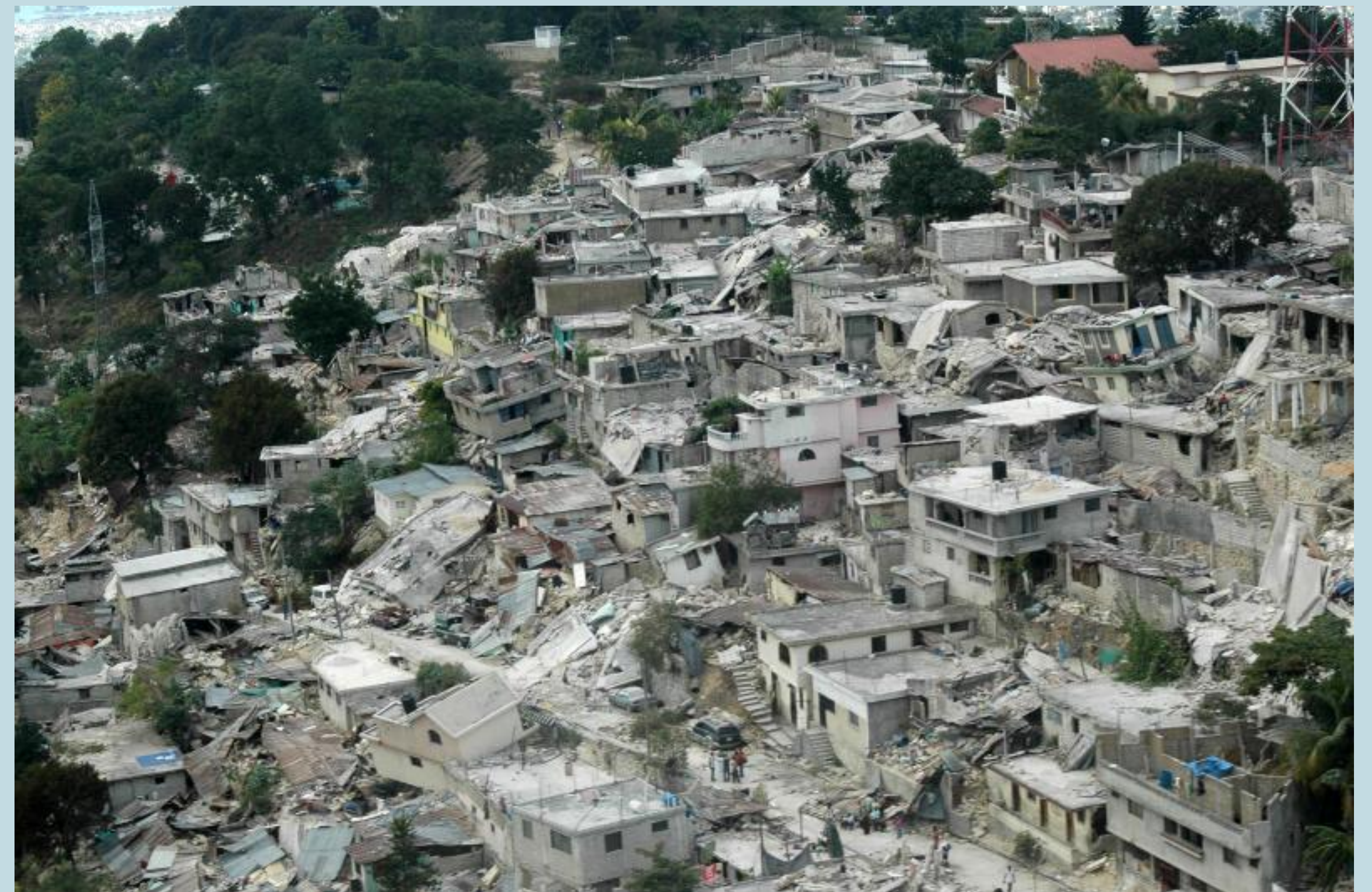
Photo taken of Haiti's capital Port-au-Prince during a joint Red Cross Red Crescent / ECHO aerial assessment mission on 13 January 2010. The devastating destruction that was caused by a 7.3 magnitude earthquake on 12 January 2010 is clearly visible.
